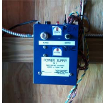
Shutter and Rotation Control Box
