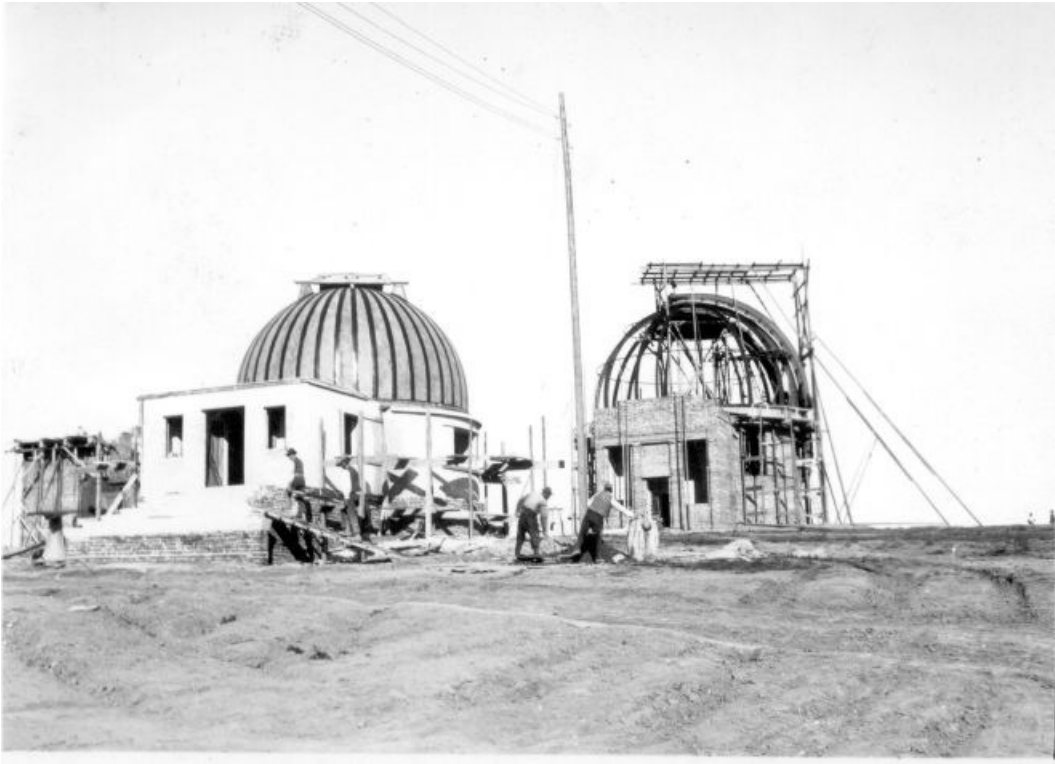
The Belgrade Astronomical Observatory under construction in 1932 on Zvezdara hill.
